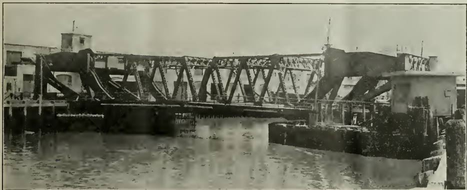
Third Street Bridge Before Demolition Began. Picture From South Side.
